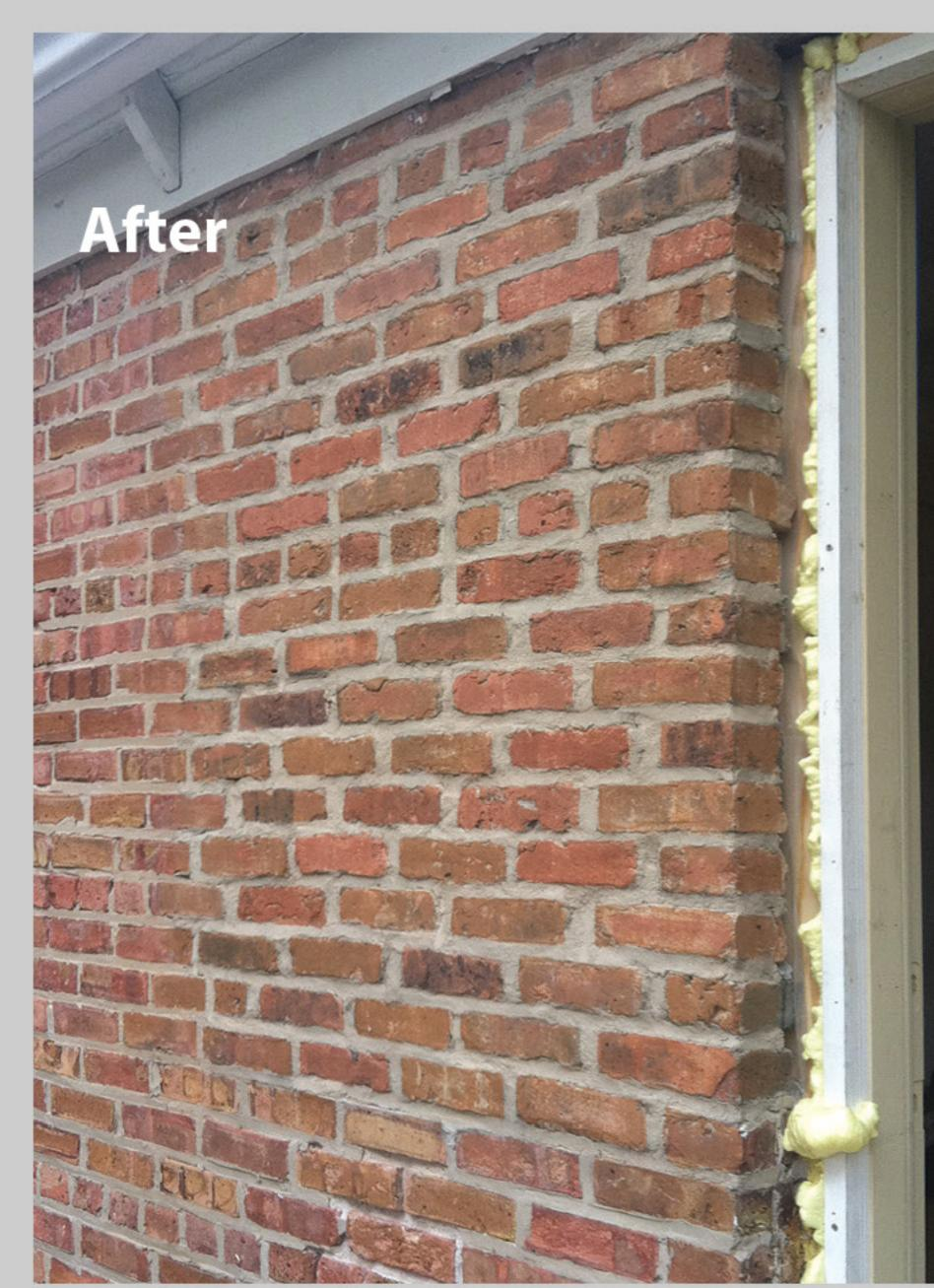
Above: The Nawkaw team helped with the selection of bricks for the repair of this column. Using bricks of the correct size, shape, and texture—even though they were a different color—was essential to achieving a precise match to the existing
